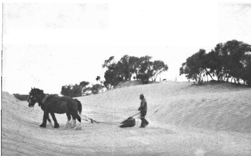
Drifting sand blocked the Calder Highway in the northern Mallee in 1945. The horses and scoop had been working for a week to open the road to the extent shown in this picture.
